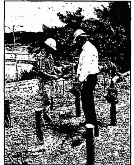
Staff members John Amerman and Bob Leonberger checking the corrosion protection level on the pipeline.
